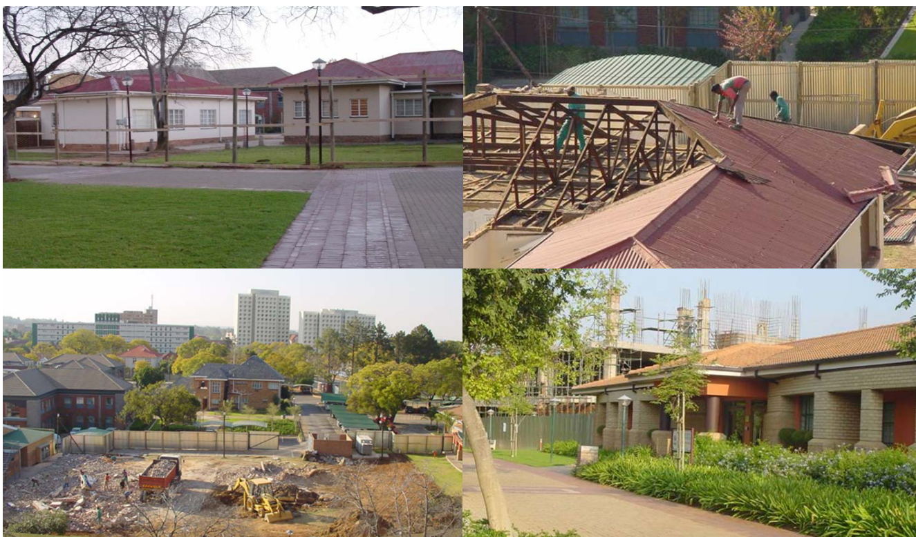
Construction of FABI Square began in 2004. This involved demolition of two houses (top).
