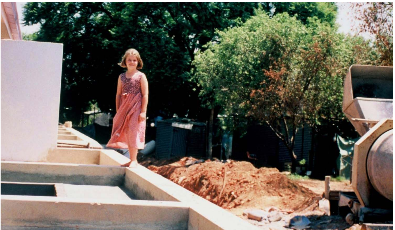
Construction of the FABI Main building began in mid 1997. The building was occupied, albeit not entirely complete, in April 1998. The girl in the picture is seven-year-old Beverley Wingfield.
